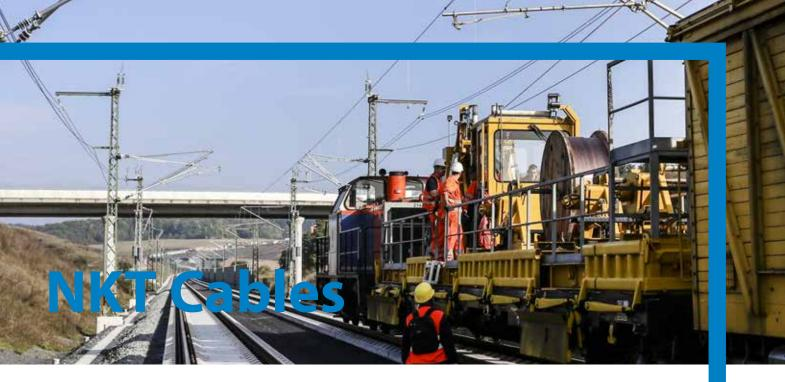
NKT Cables' railway contact wire is being installed on the high-speed line Berlin-Munich, Germany. Trains will run up to 330 km/h and shorten the travelling time from 6 to 4 hours.
