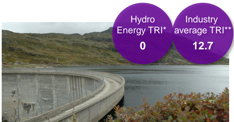
Reservoirs and dams
