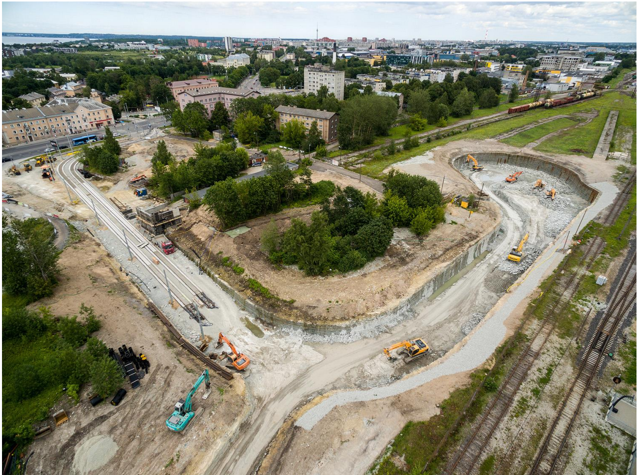
EXTENSION OF THE TRAM TRACKS AND CONSTRUCTION OF A TRAM TURNAROUND LOOP ON THE PETERBURI ROAD 2 PLOT UNDER THE CONTRACT TO DESIGN AND RENOVATION OF THE INFRASTRUCTURE OF TALLINN TRAM LINE NO. 4 BY A CONSORTIUM CONSISTING OF AS MERKO EHITUS EESTI, KMG INSENEREHITUSE AS AND RATATEK OY.
