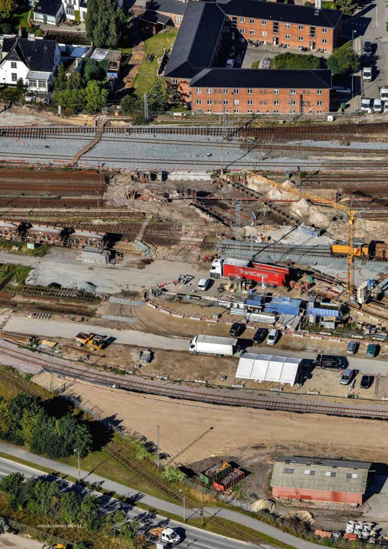
SE II WE and the AR m 4 I. 11 2 1111 Ante RE . Jan de Carto 1 NS IN 32 1 -1 (j) 1.00 W. In Køge, Aarsleff and the subsidiary Aarsleff Rail A/S con-struct a tunnel which will lead the traffic under 11 tracks at the station and connect the port with the city centre. 3 ~
