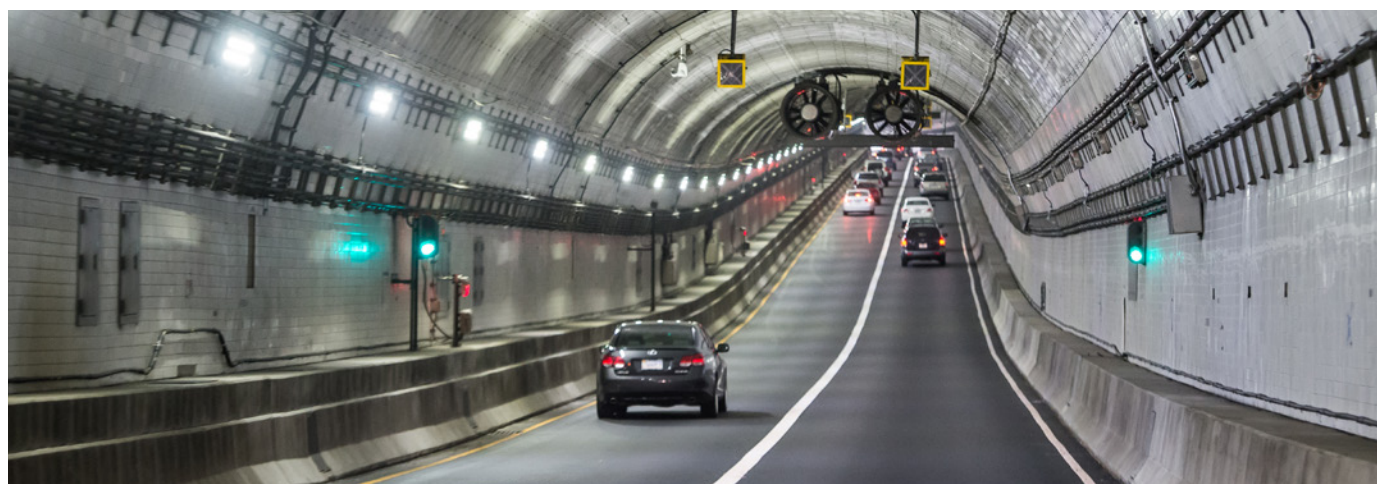
Elizabeth River Tunnels, Virginia, U.S.
