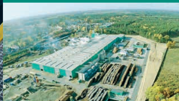
Steico's new LVL mill in Czarna Woda, Poland
