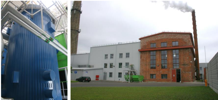
Photo: new biofuel boilers and renewed Inkaras boiler-house building
