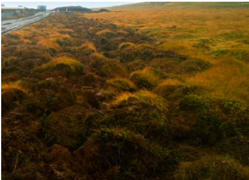
Figure 5b. The turf was placed over the ditch to utilise the native vegetation. Thus biodiversity can be maintained, while enhancing the visual impact and effective land reclamation. Photograph: Magnea Magnúsdóttir.
