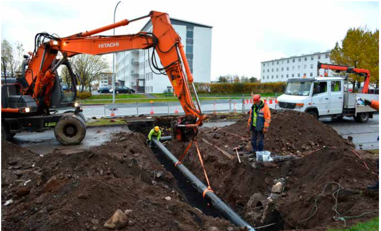
Figure 13. Work on water pipeline on Kringlumýrarbraut in Reykjavík. Photograph: Hildur Ingvarsdóttir.
