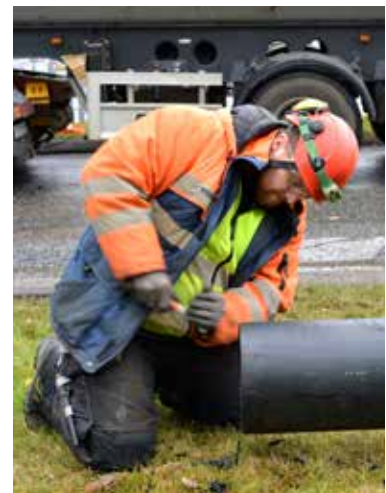
Figure 2. Working on a water supply pipeline in Reykjavik. Photograph: Hildur Ingvarsdóttir.
