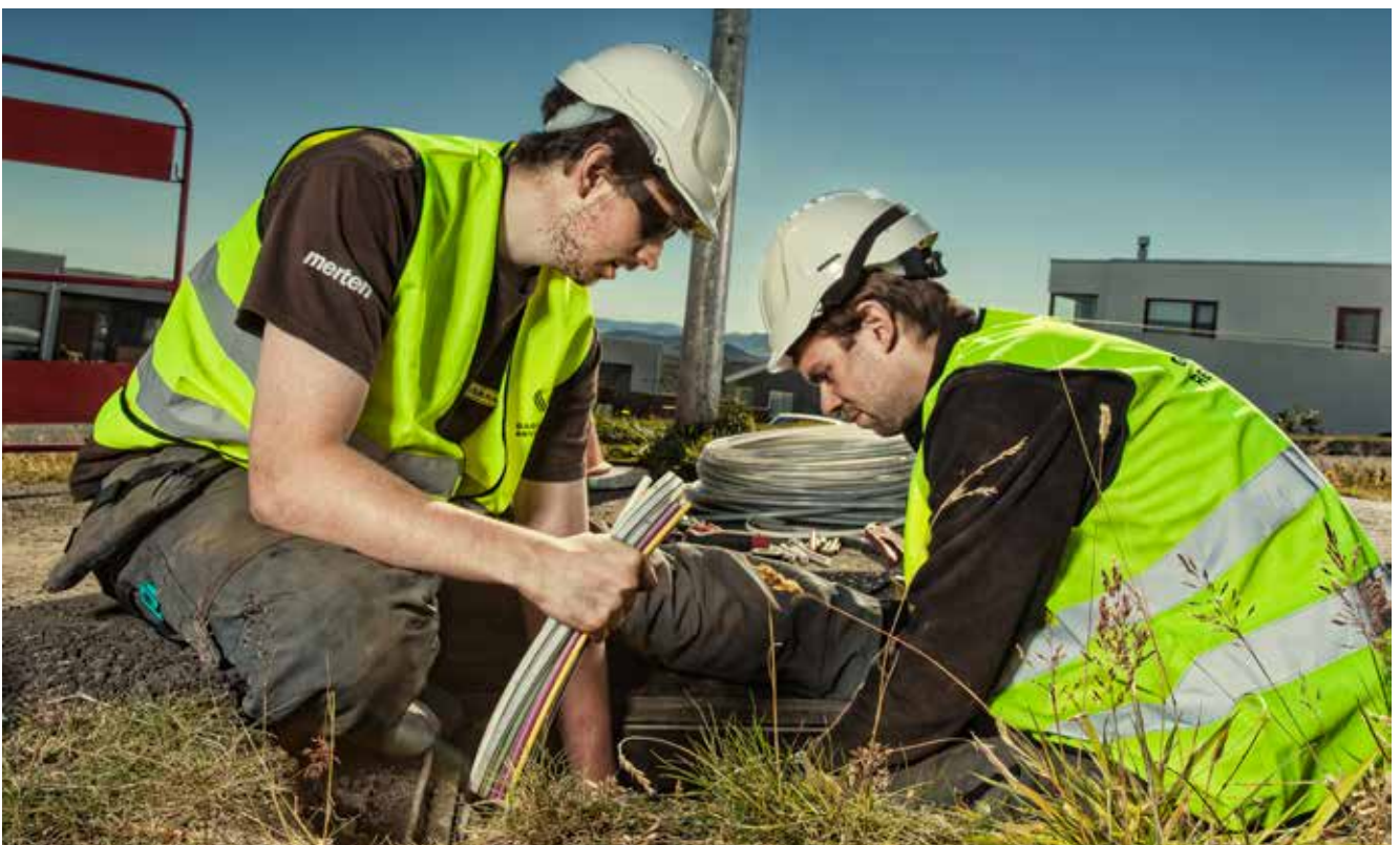
Figure 15. Laying fibre optic cables in Hafnarfjörður. Photograph: Sigurjón Ragnar.
