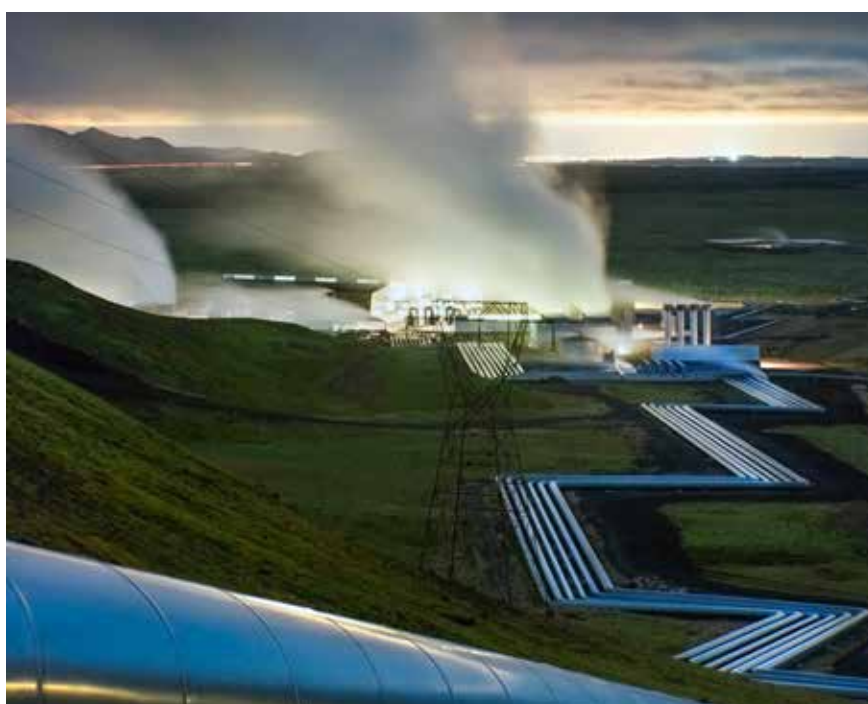
Figure 8. Hellisheidi Geothermal Power Plant. Photograph: Gunnar Svanberg.
