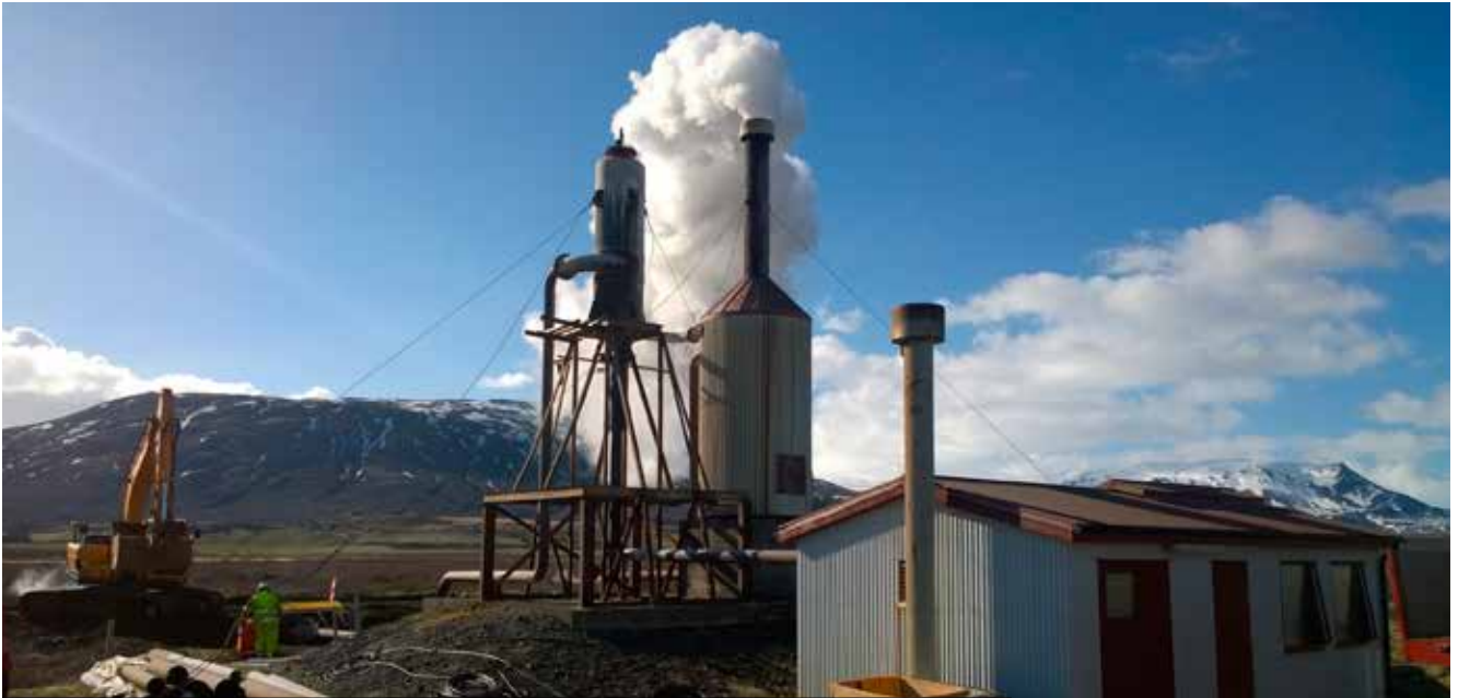
Figure 11. Changing well head in Efri-Reykir. Photograph: Guðmundur Óli Guðmundsson
