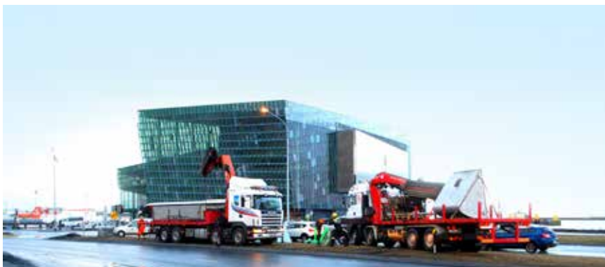
Figure 26. Installation of a new emergency outlet valve at a pumping station on Ingólfsstraeti in Reykjavik. Photograph: Hildur Ingvarsdóttir.
