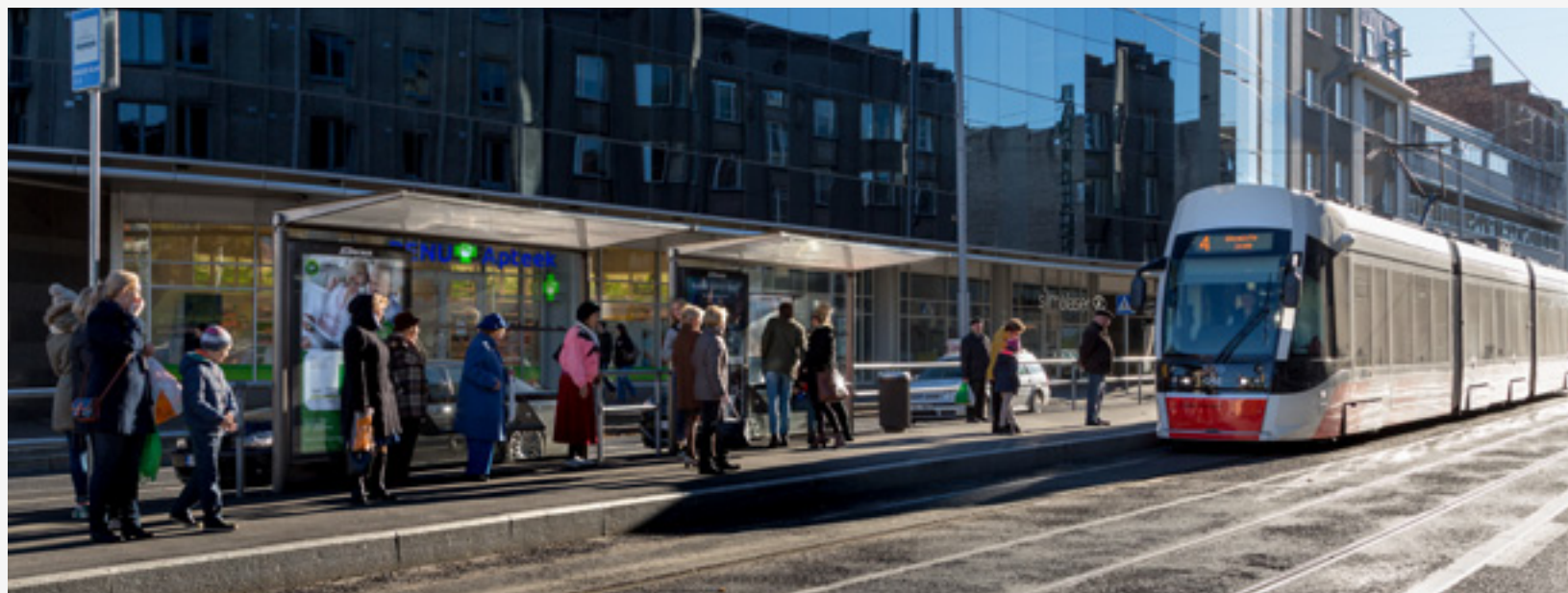
AS A RESULT OF THE DESIGN AND RENOVATION OF THE INFRASTRUCTURE OF TALLINN TRAM LINE NO.4, THE PEOPLE IN TALLINN ARE SERVED BY THE NEW TRAMS.
