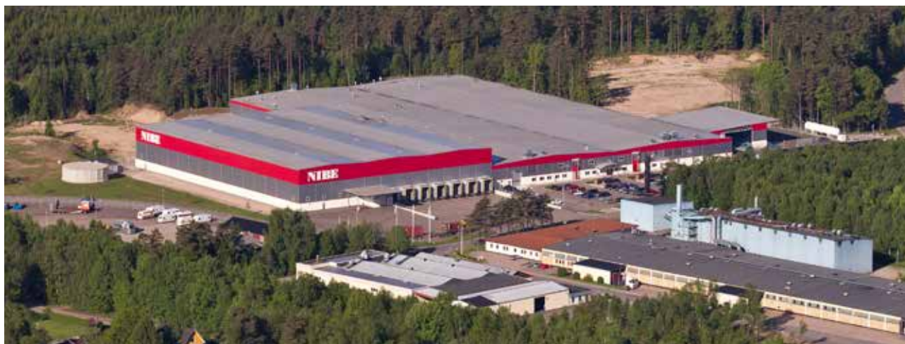
The production plant in Markaryd, Sweden, primarily manufactures sheet steel stove products and complete chimney systems for the brands Contura and Premodul by Contura. The rate of production was increased considerably during the first half of the year to meet an expected increase in demand and guarantee both good delivery capacity and high delivery reliability for the coming peak season during autumn and winter 2016.
