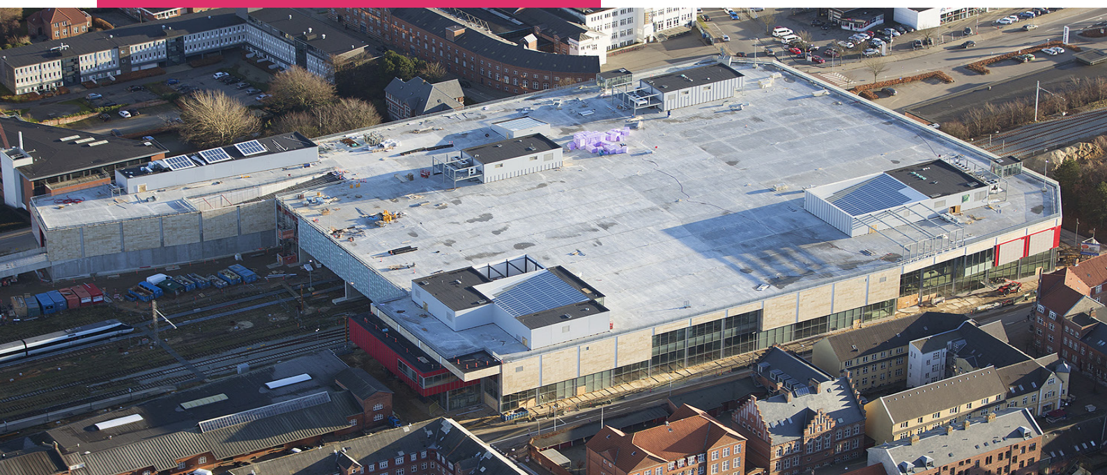
BROEN Shopping, Esbjerg, Denmark - scheduled for completion in April 2017
