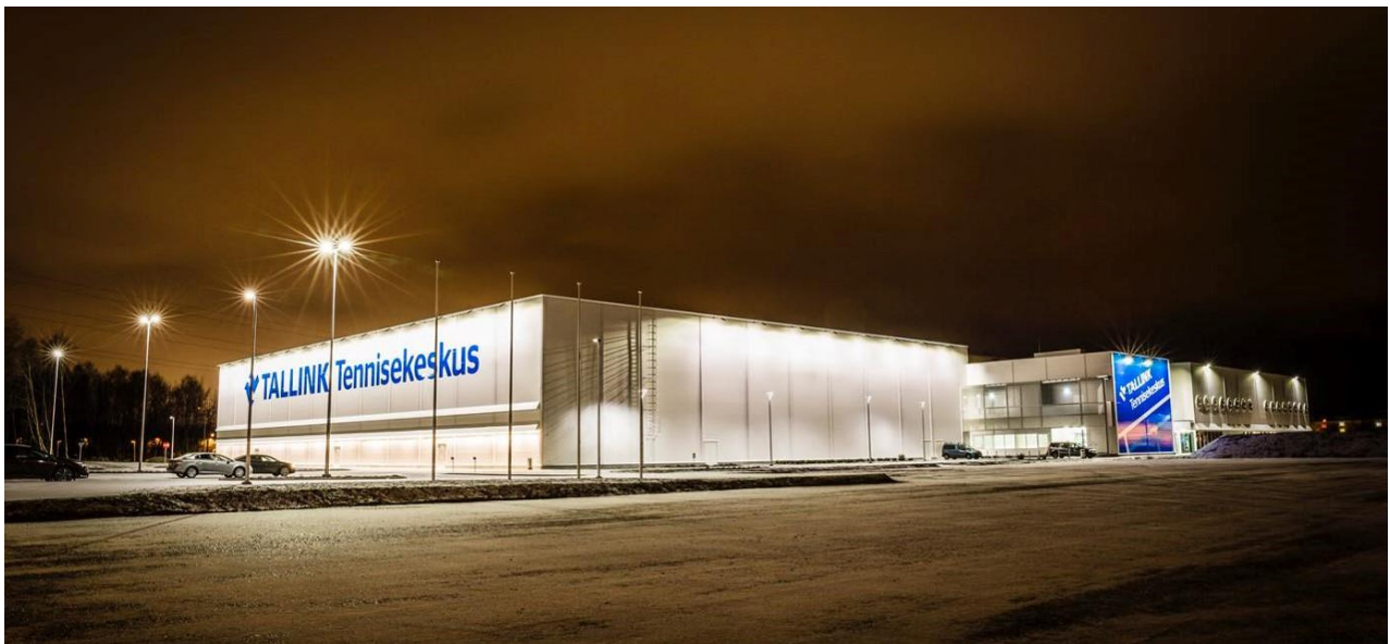
COMPLETED IN Q4, TALLINK TENNIS CENTRE IN LASNAMÄE DISTRICT OF TALLINN INCLUDES 14 TENNIS COURTS, 10 BADMINTON COURTS, GYM, FITNESS HALLS AND ADMINISTRATION ROOMS.
