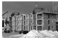
Residential Construction Tuujuk Nuuk
