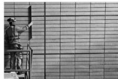
Interior works Cph Metro Copenhagen
