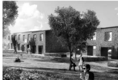
Residential refurbishment Ryhaven Aarhus
