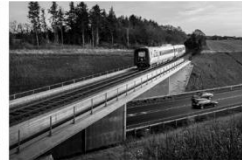
Construction and refurbishment of 56 bridges Banedanmark Copenhagen-Rødby
