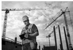
Construction of shell structure Nyt Aalborg Universitetshospital Aalborg
