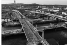
Construction of bridge in joint venture Marieholm Broen Gothenburg
