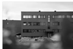
Residential Refurbishment Langkærparken Aarhus
