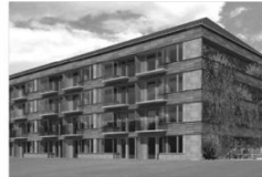
Residential refurbishment Korngården Ballerup
