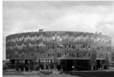
Construction of school Kalvebod Fælled Skole Copenhagen
