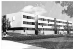
Residential Refurbishment Åbyhøjgård Aarhus
