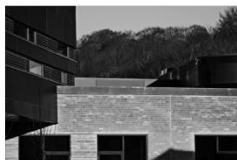
Construction of psychiatric ward on PPP basis Vejle Sygehus Vejle
