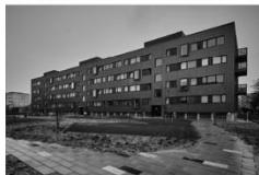
Residential Refurbishment Rosenhøj Viby
