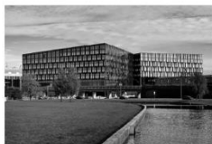
Construction of head office Nordea Ørestaden
