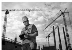
Construction of shell structure Nyt Aalborg Universitetshospital Aalborg
