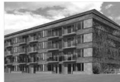
Residential refurbishment Korngården Ballerup
