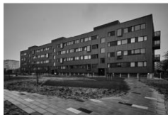
Residential Refurbishment Rosenhøj Viby
