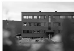
Residential Refurbishment Langkærparken Aarhus
