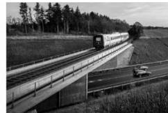
Construction and refurbishment of 56 bridges Banedanmark Copenhagen-Rødby
