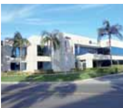
CAVOTEC DABICO/INET Cypress, CA, USA
