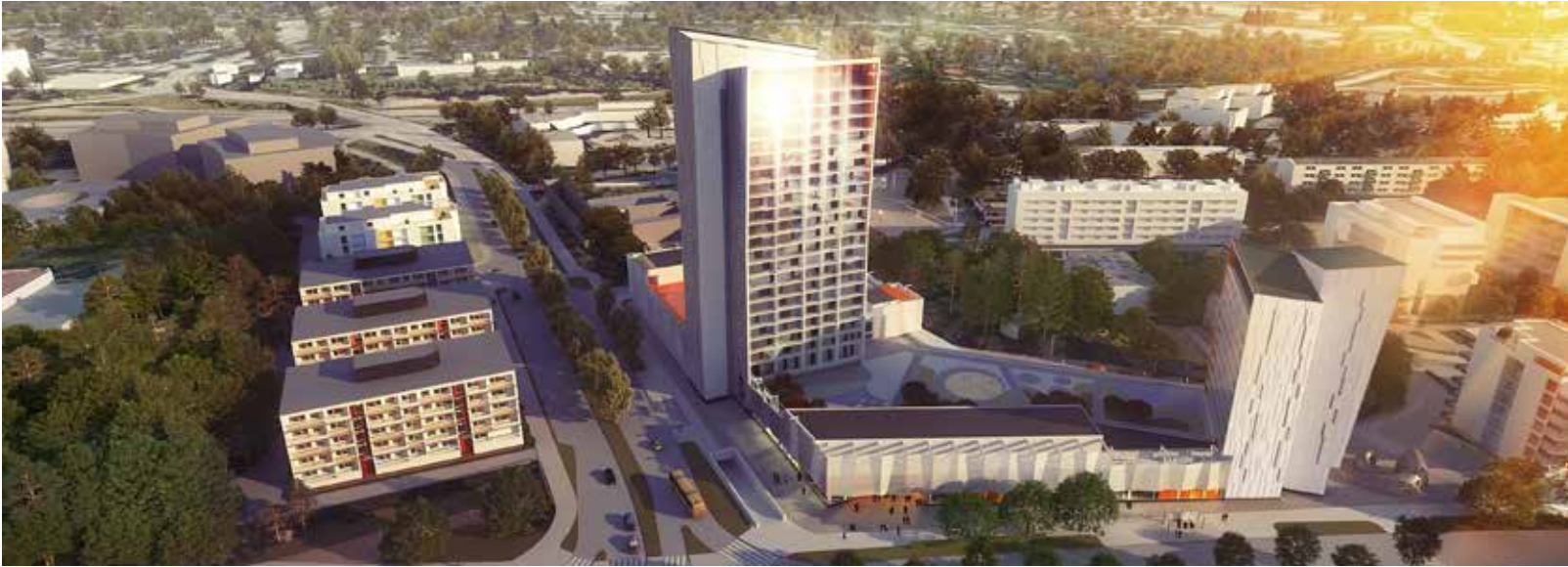
A modern Metro Centre, the Niitty shopping centre meadow and homes for thousands of new residents will be built at Niittykumpu, Espoo.
