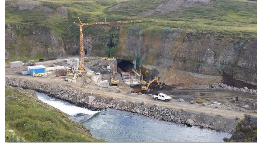
Intake facility at Laxarvirkjun 3
