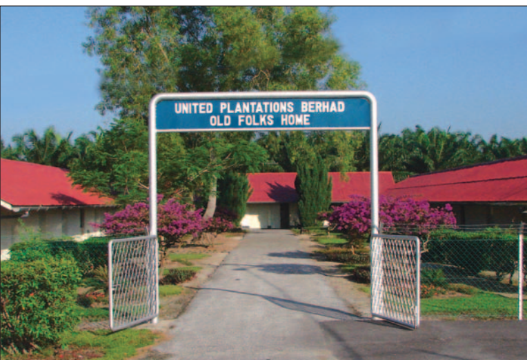
A front view of the Old Folks Home in Jendarata Estate equipped with the best possible facilities for our retired and aged workers. A full time caretaker is employed to ensure that they get the best possible care and attention at all times.
