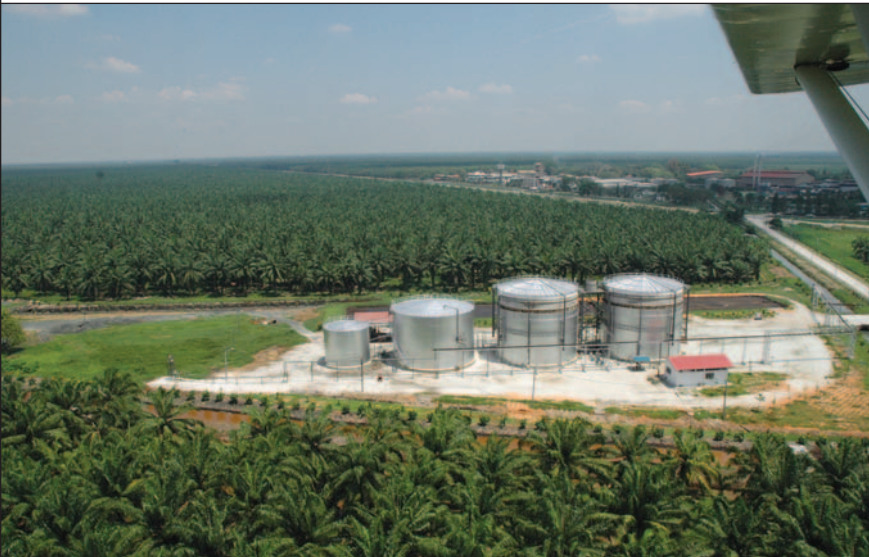
An aerial view of the Biogas Digester at Jendarata Estate which is certified as a Clean Development Mechanism Project enabling the mill to generate biorenewable energy from the Palm Oil Mill effluent.
