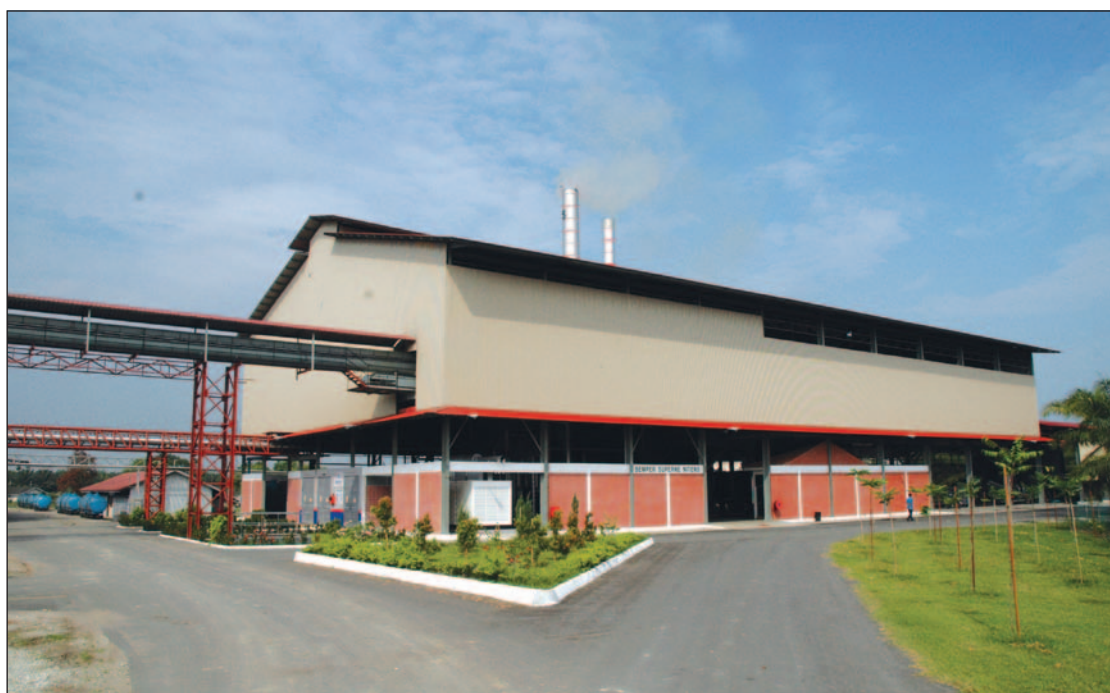
Clean air emissions from the new Biomass Reciprocating Boiler at Jendarata Estate Palm Oil Mill
