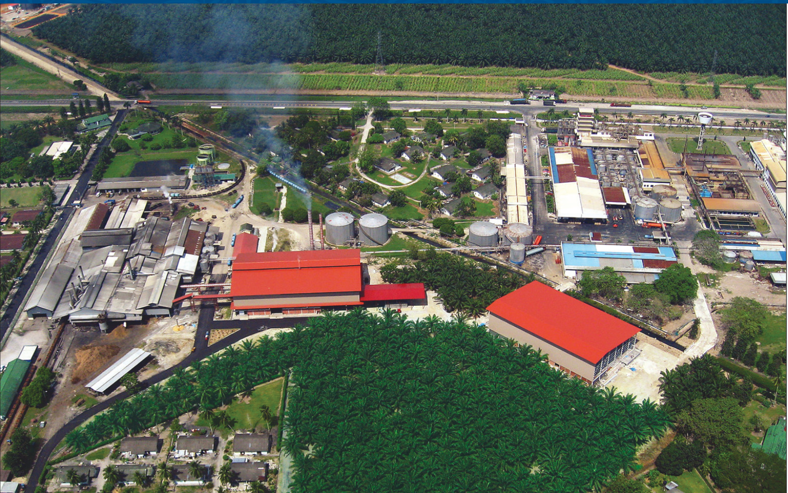
An aerial view of the state of the art Biomass Reciprocating Boiler (BRB) at the Jendarata Palm Oil Mill Complex. The project is certified as a Clean Development Mechanism Project in accordance with the Kyoto Protocol with the objective to reduce Green House Gas Emissions. The building to the right of the BRB is Unitata's new warehouse which caters for its finished products. On the top right hand corner, the Unitata Refinery Complex can be seen.
