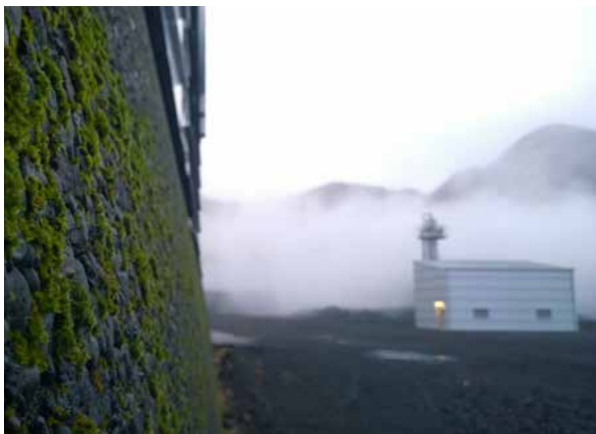
Moss on the walls of the powerstation at the Hellisheidi Geothermal Power Plant and the hydrogen sulphide abatement unit in the background. Photograph: Magnea Magnúsdóttir.
