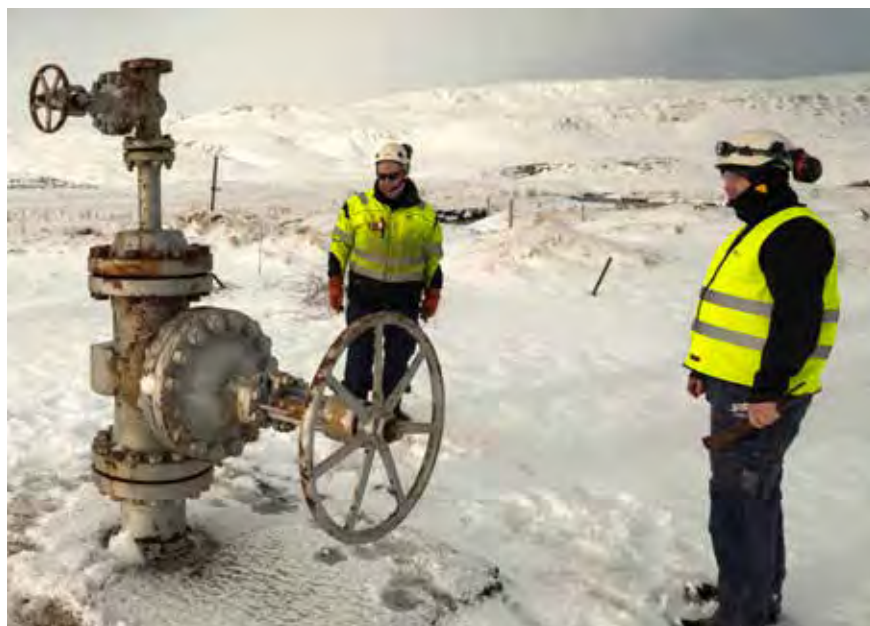
Working on a hot water utility in Hveragerði. Photograph: Gretar Ívarsson.
