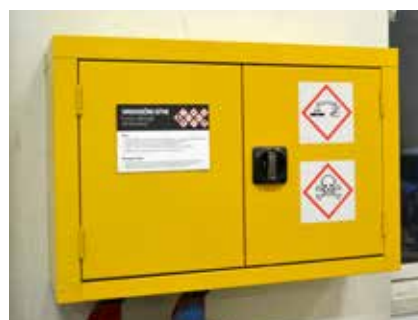
A new and labelled cabinet for acids was installed at the Veitur Utilities workplace in Bæjarháls in 2016. Photograph: Unnur Jónsdóttir.
