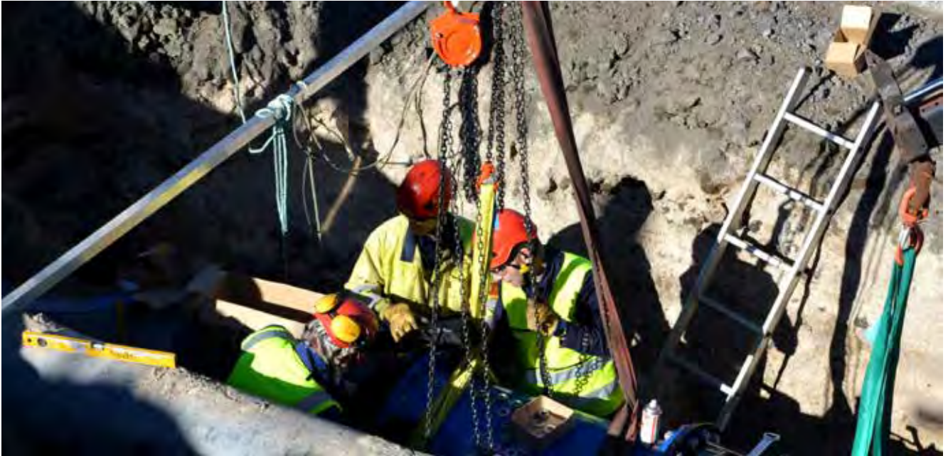
Working on the water supply pipeline in Reykjavík. Photograph: Hildur Ingvarsdóttir.
