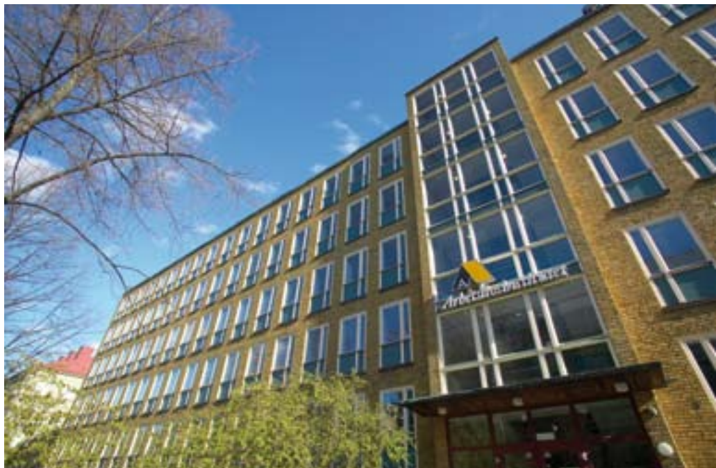
Mimer 5 with about 12,000 sq.m lettable space was acquired in February 2007. The property strengthens the portfolio in the Norrtull/Norra station-area.
