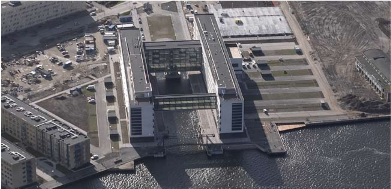
Corporate headquarters for KMD, Aalborg, Denmark At end-2006, the 26,000 m 2 corporate headquarters building was handed over to KMD (Kommunedata).
