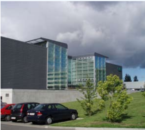
CMC, Vandtårnsvej, Copenhagen, Denmark This 8,300 m 2 project has been sold and handed over to a Luxemburg fund.
