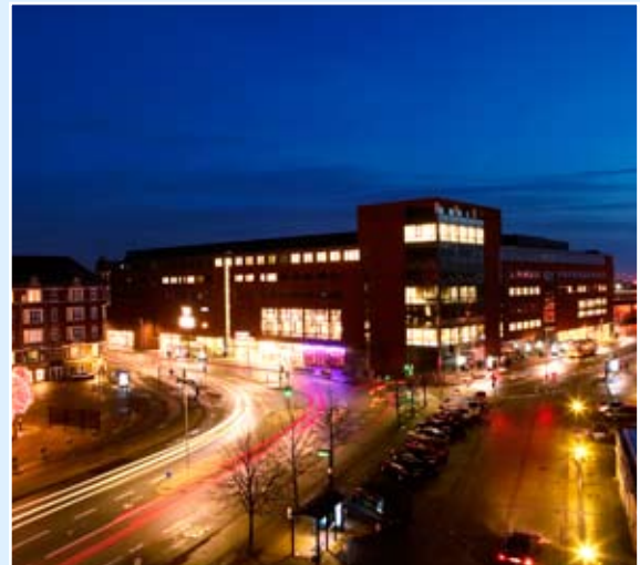
The Kennedy Arcade, Aalborg, Denmark This 29,000 m 2 project, exclusive of the cinema section, was sold and handed over to Aberdeen Property Investors in the past financial year.
