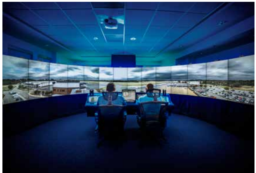
Saab's Remote Tower air traffic control system installed at Leesburg Airport in the US.
