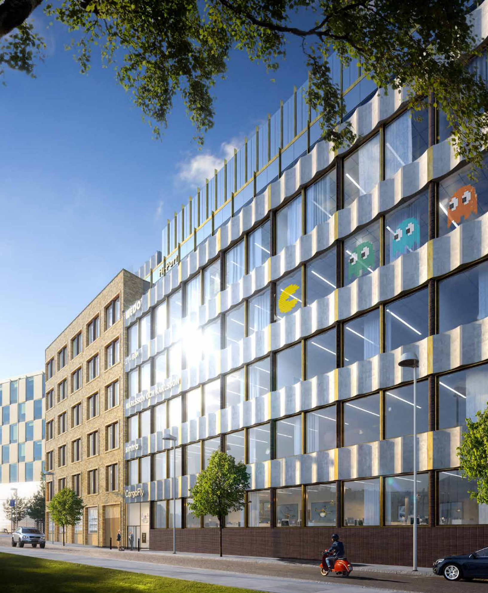
The Postterminalen 1 property in Lund consists of two separate buildings; Posthornet and Frimärket. The names inspired the design of the facades, which were designed by architect Charlotte Von Brömssen at Tengbom.
