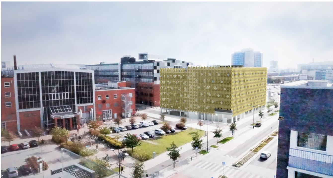
Allow us to present Hordaland 1, the new multistorey car park in Dockan, Malmö. The 15,000 m 2 multistorey car park will be completed in autumn 2017.
